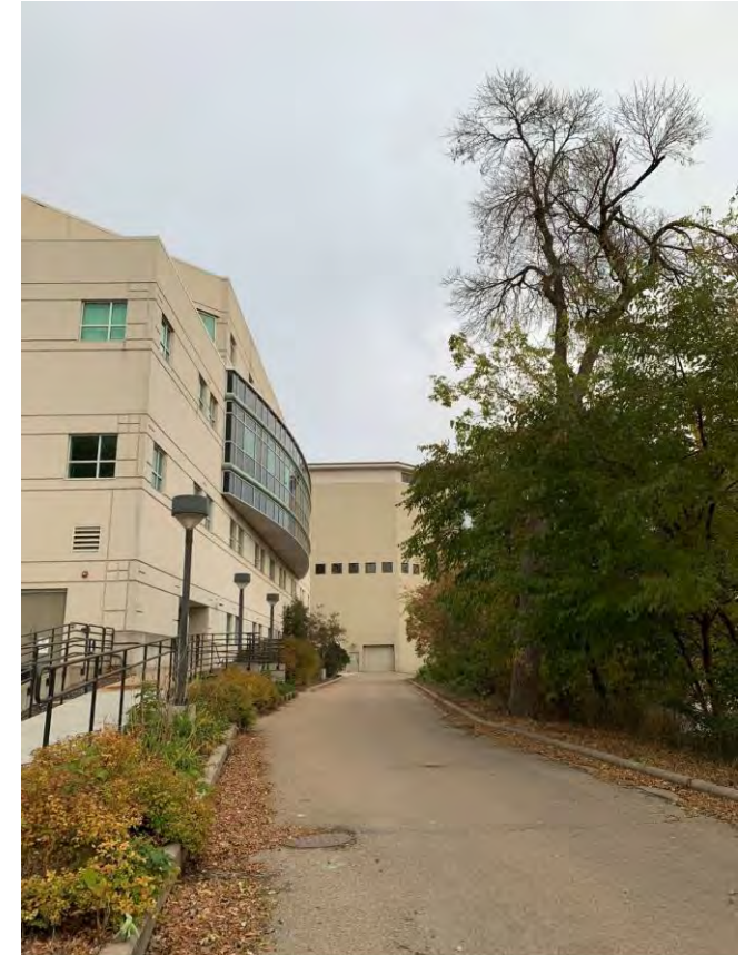
Back Entrance: 1 st floor, along the river The rounded windows are Psychology offices
